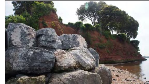
Rock armour protecting eroding headland, Exe Estuary
